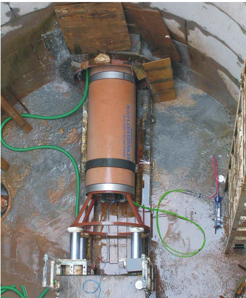
DN700 SLIPLINING, CARDIFF
