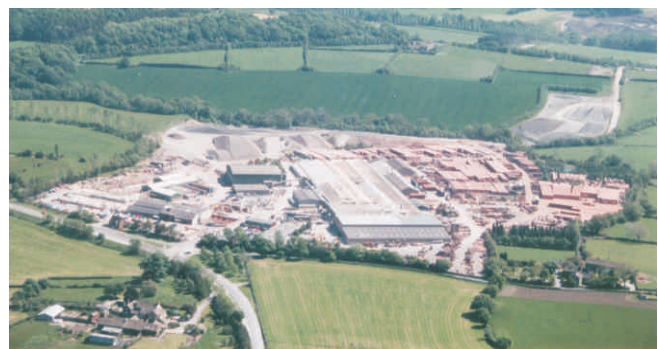
South Yorkshire site.
